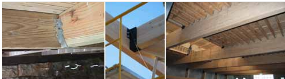
Figure 8-28. Typical joist hanger connectors.
